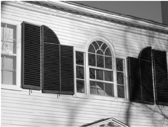
Detail of Daniel Johnston house (1805) on Main Street with original shutters including hinged pair for Palladian window. Note interior shutters in left window. Author's photograph.
