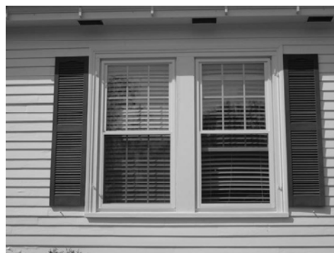
"Faux shutters" are screwed onto siding rather than suspended from pintles. Author's photograph.
