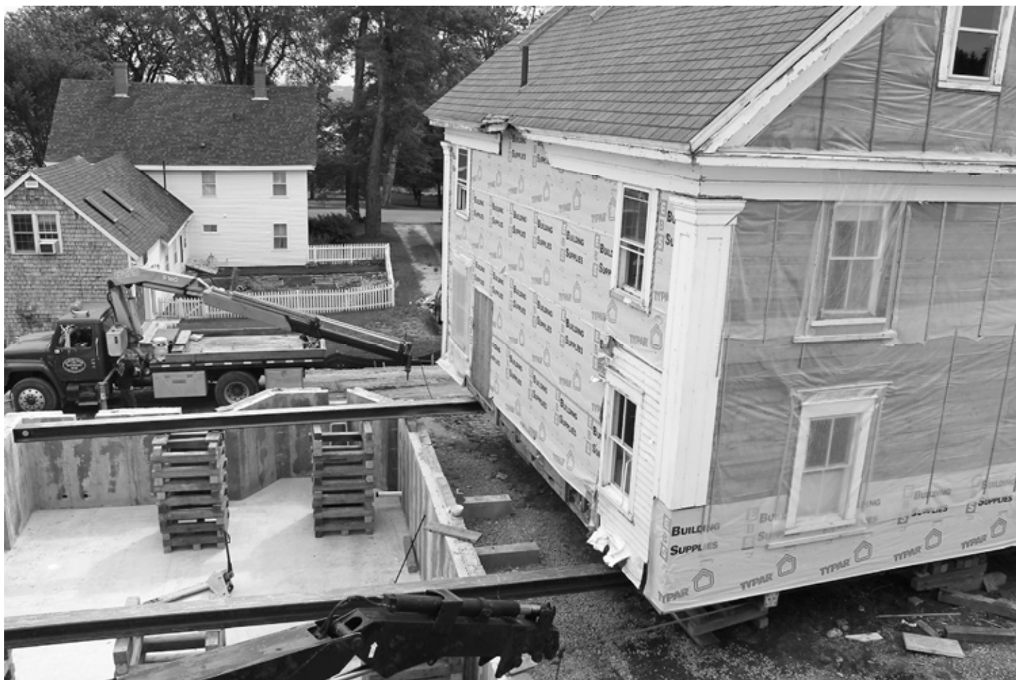
Sliding onto the new foundation. September 10, 2013
